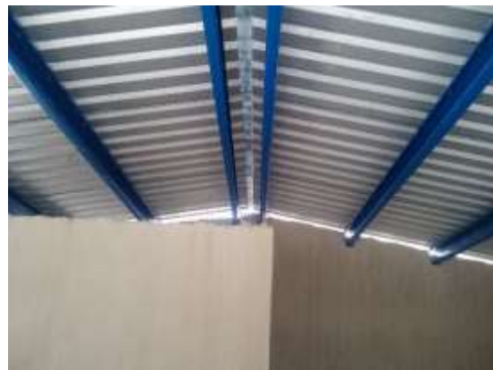
Techumbre vista interior
